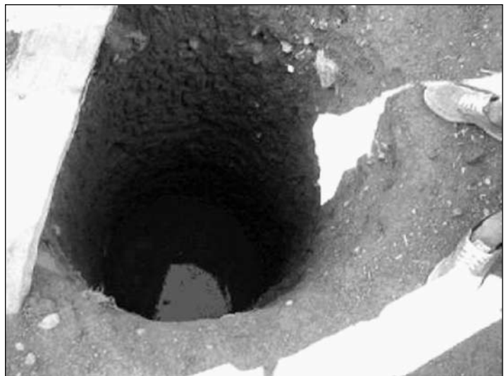
Figure 2: Cha (harvesting snow in wells) in Ghor
